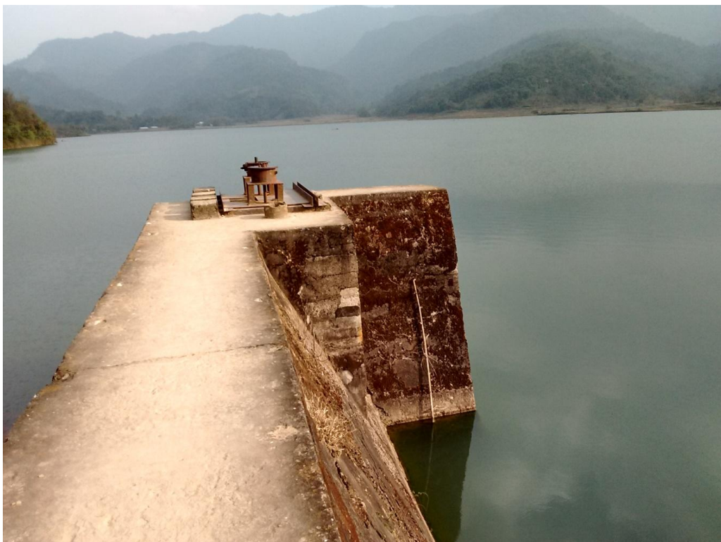
Fig.14: Intake structure showing outlet gates for water discharge for irrigation
