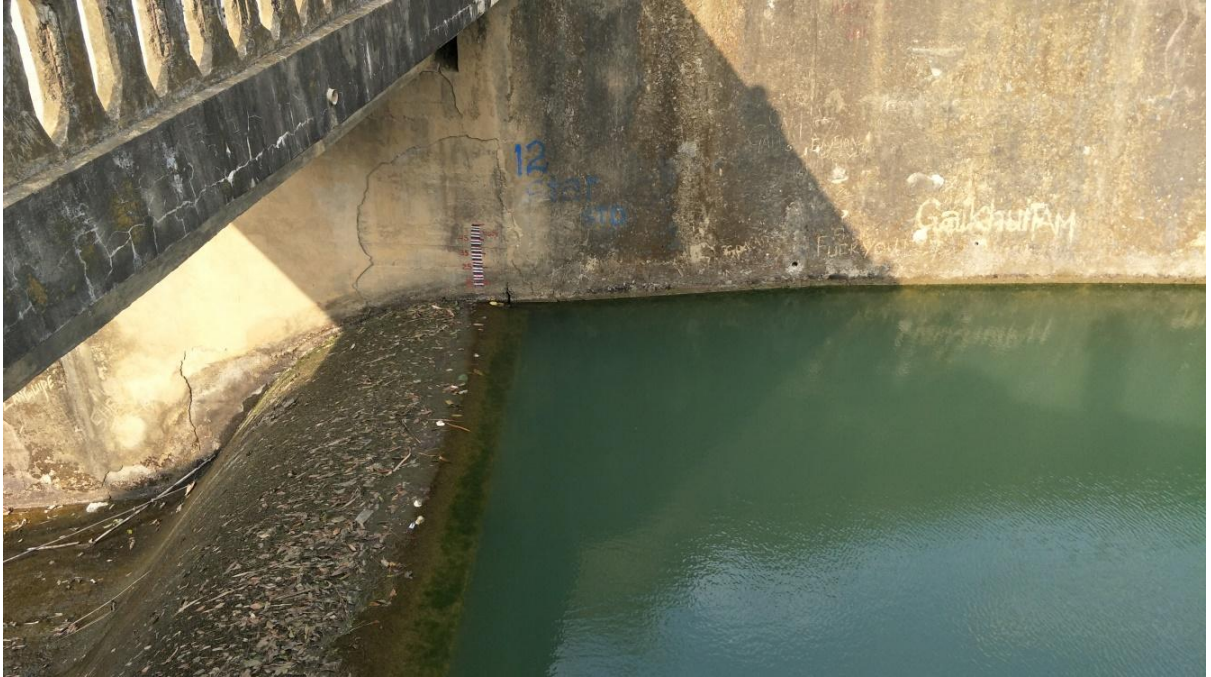
Photo 13: Crest of spillway with Water level marking
