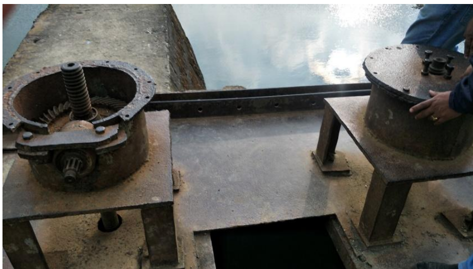
Fig.15: Locked gates for regulating the discharge to canals
