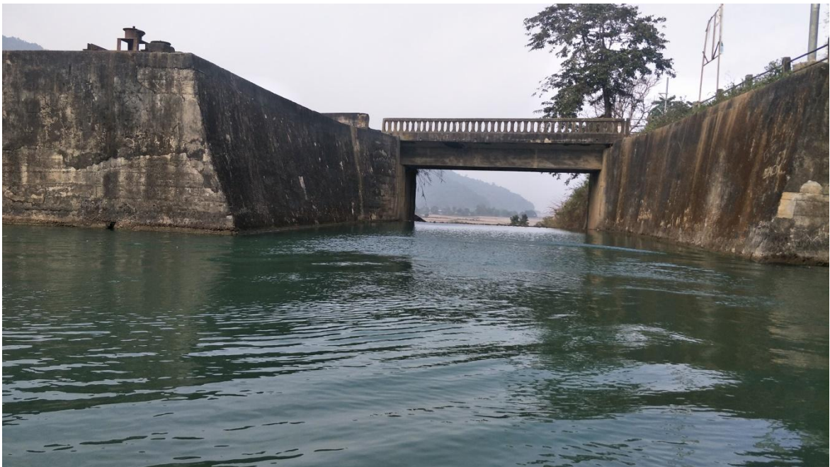
Photo 4: Spillway of Khoupum dam
